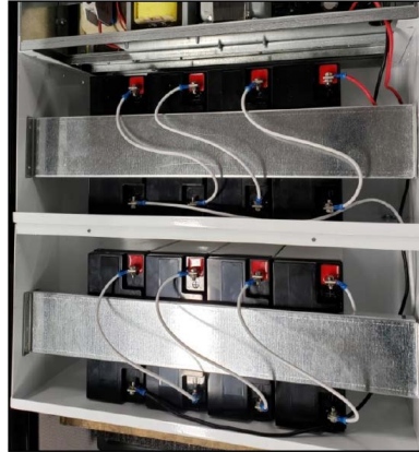
Battery brackets installed on the front
